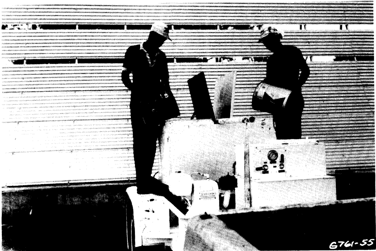
Figure 5-3. Cold-Applied, Two-Component Sealant Application Equipment.
